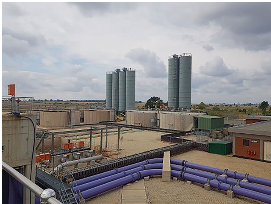
Fig. 4.7 Silos filled with lime. (Photograph by researcher)
